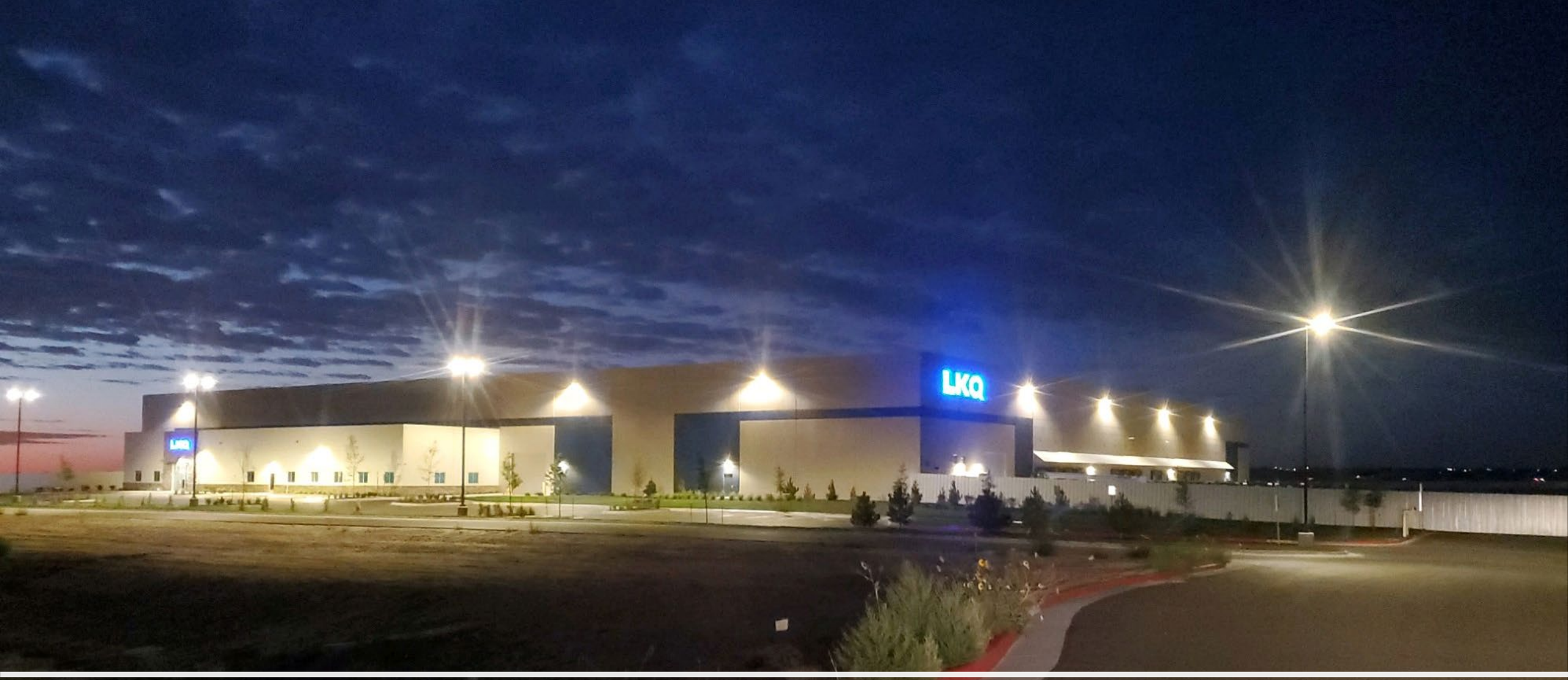
New LKQ Facility in Denver CO (Completed in 2022)
